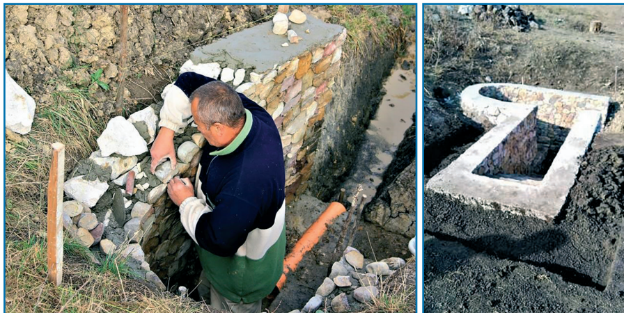
Figure 22. Unclogging and arrangement of springs
